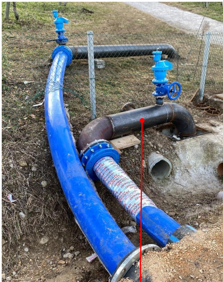
Bypass tie-in point with existing line
