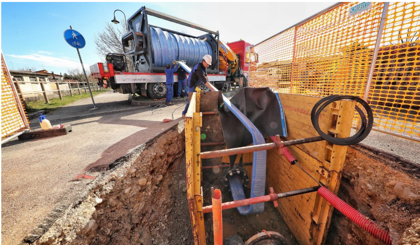
Line rehabilitation during bypass operation
