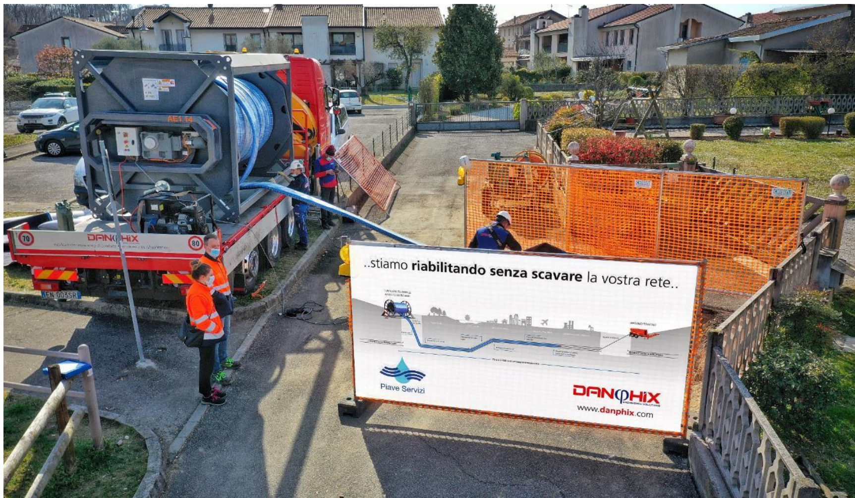
Line rehabilitation during bypass operation
