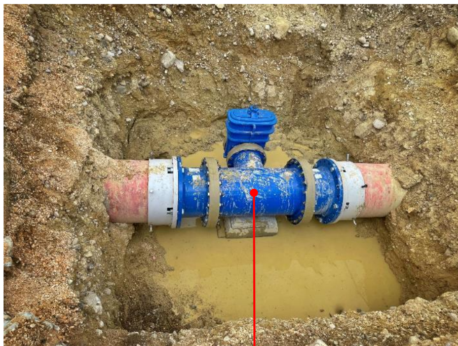
DN300 branch connection restored
